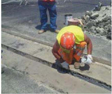
Photo 5 Coating the concrete faces
