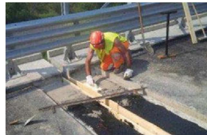
Photo 4 Levelling of the elements
