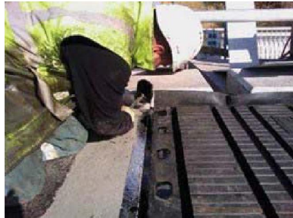
Photo 8: Filling in the transition zone
