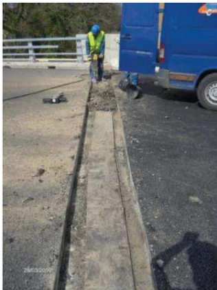
Photo 1: Removing and restoring the concrete support.
