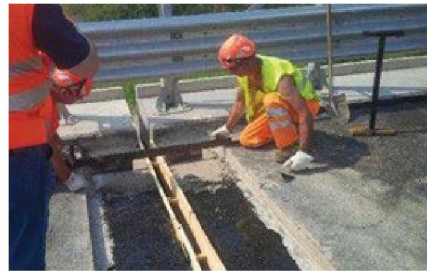
Photo 3 Setting the bedding thickness by the JIG
