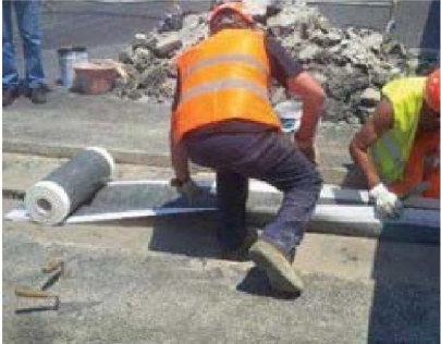
Photo 6 Membrane installation
