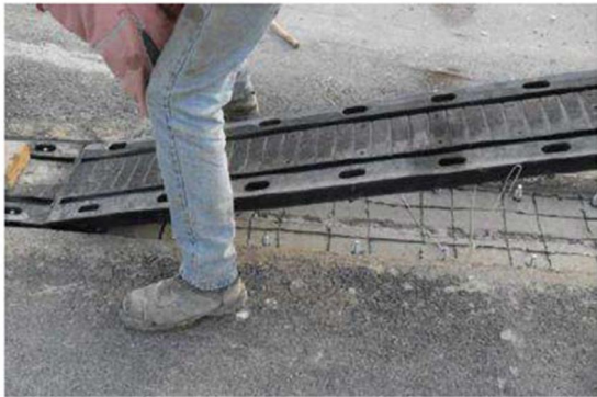
Photo 7: Installation of joint elements
