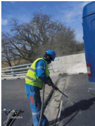
Photo 2: Clean the concrete support and the joint gap.
