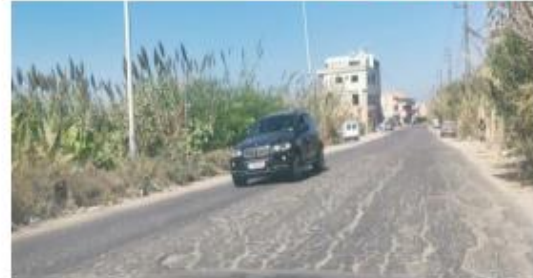
Moderate to Severe alligator cracks in the
