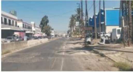
Poor Asphalt repair, and sunken utility trench
