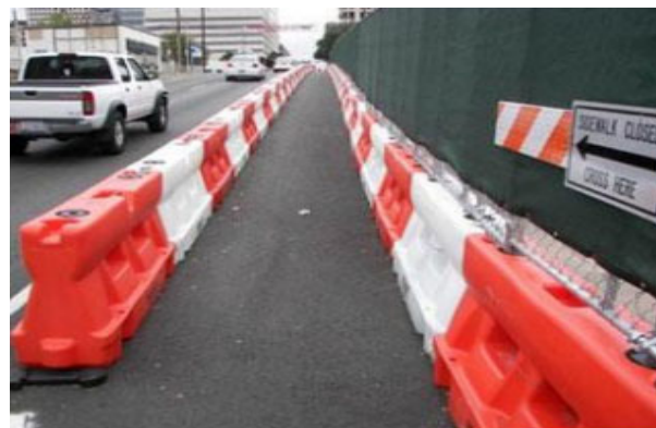
Figure 9-15: Plastic Water filled Barricades within Work Zone.
