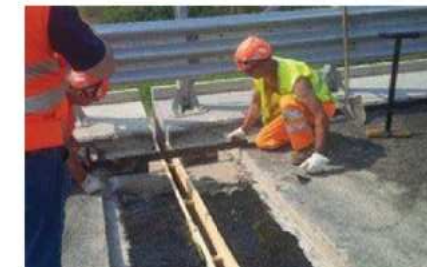
Photo 3 Setting the bedding thickness by the JIG
