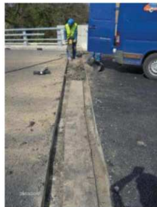
Photo 1: Removing and restoring the concrete support.
