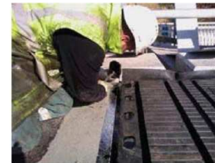
Photo 8: Filling in the transition zone
