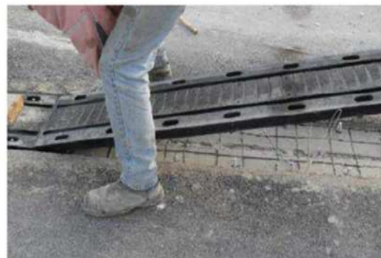
Photo 7: Installation of joint elements
