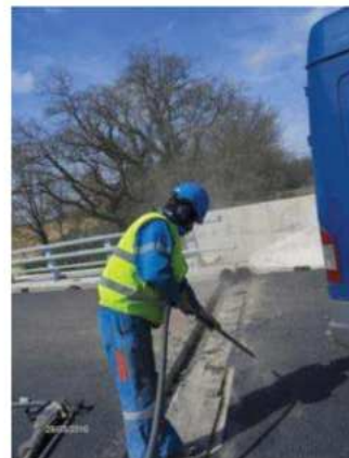
Photo 2: Clean the concrete support and the joint gap.
