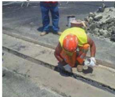
Photo 5 Coating the concrete faces
