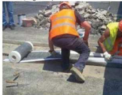
Photo 6 Membrane installation
