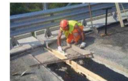
Photo 4 Levelling of the elements
