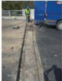
Photo 1: Removing and restoring the concrete support.
