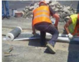
Photo 5 Coating the concrete faces
