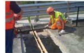
Photo 3 Setting the bedding thickness by the JIG
