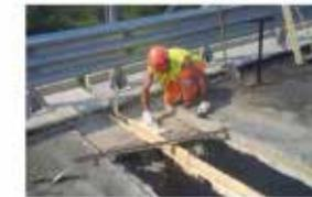
Photo 4 Levelling of the elements
