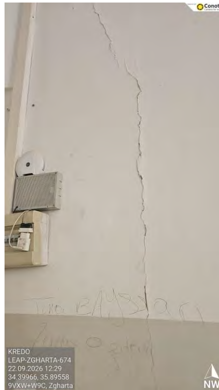
Figure 8 - Wall Cracks
