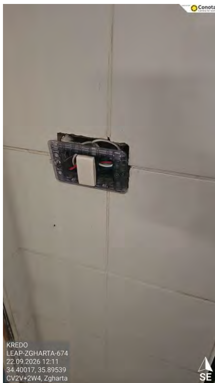
Figure 13 - Damaged socket
