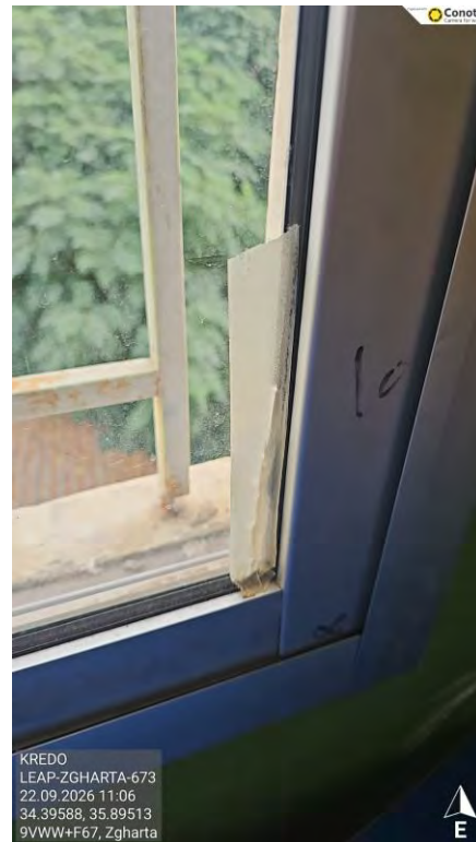
Figure 12 - Cracked Glazing
