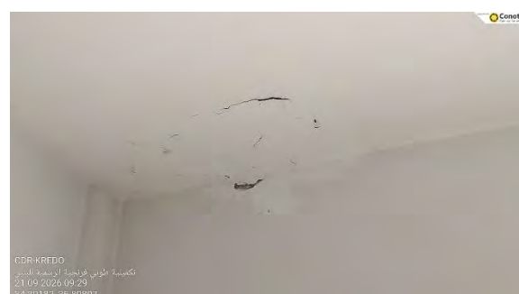
Figure 10 - Damaged Plaster
