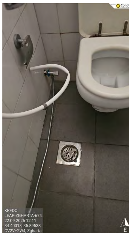
Figure 16 - Damaged Bidet
