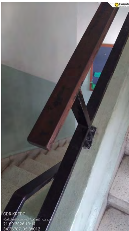
Figure 10 - Rusted Handrail
