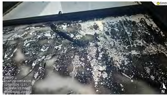
Figure 12 - Cracked Glazing
