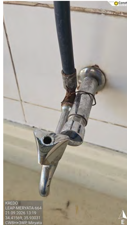
Figure 12 – Damaged Taps
