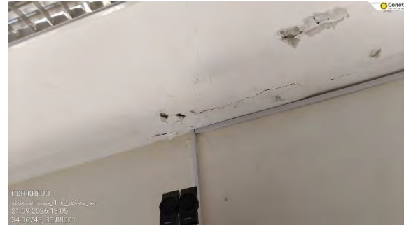
Figure 13 - Damaged Plaster
