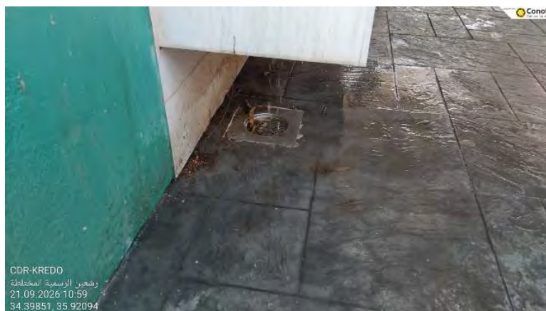
Figure 20 - Removed Drinking Basin Drainage
