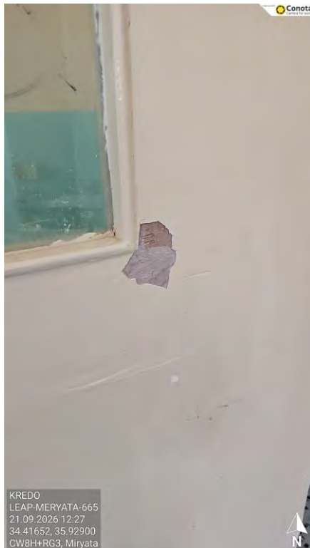
Figure 7 – Damaged Door
