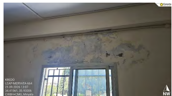
Figure 10 - Water Leakage
