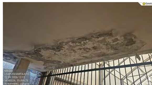
Figure 10 - Water Leakage
