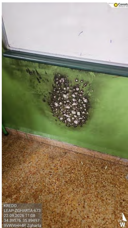
Figure 9 – Damaged Paint
