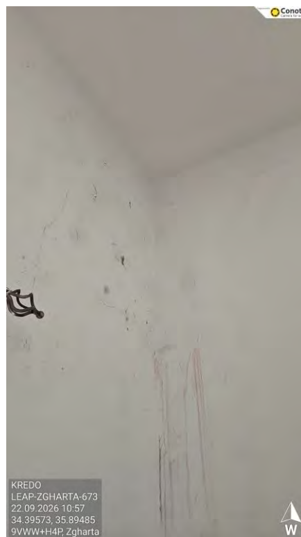
Figure 10 - Water Leakage
