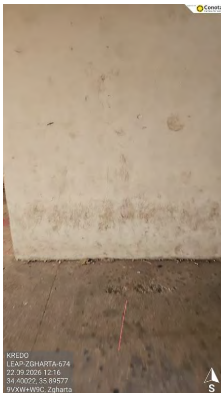
Figure 9 - Damaged Paint
