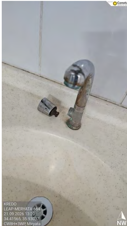
Figure 11 – Damaged Mixers
