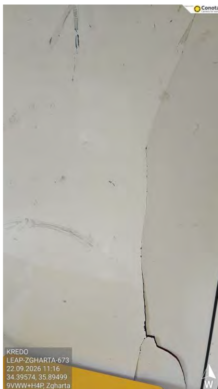
Figure 13 – Damaged Plastering
