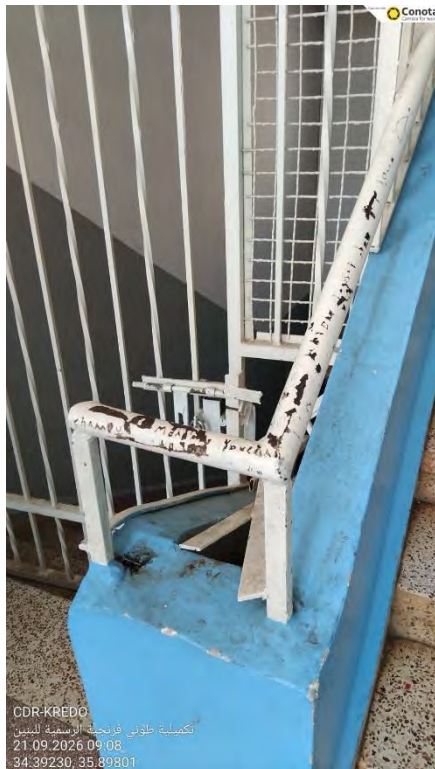
Figure 17 - Rusted Handrail
