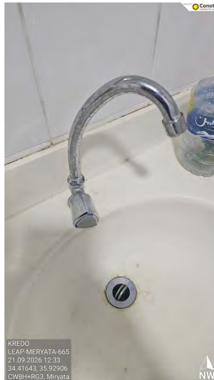
Figure 8 – Damaged Mixers
