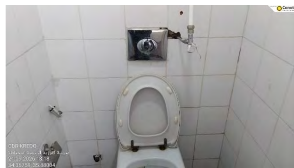
Figure 7 - Leaking Flusher
