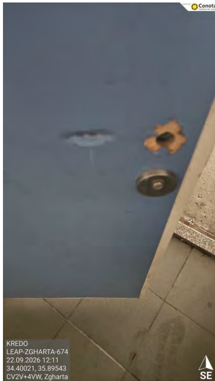
Figure 7 – Damaged Door
