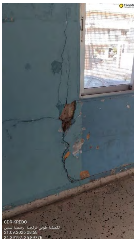
Figure 19 - Damaged Plaster
