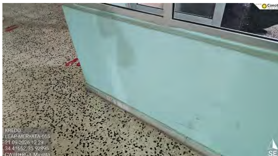
Figure 11 – Damaged Paint
