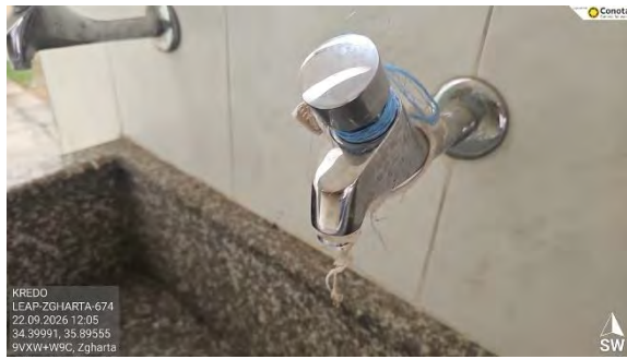
Figure 11 - Damaged Tap
