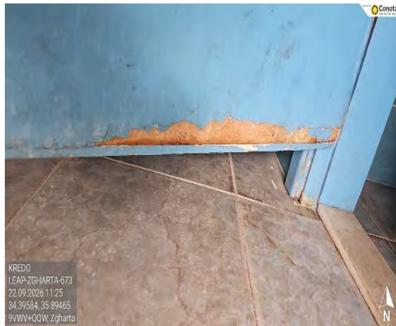
Figure 19 - Damaged Doors
