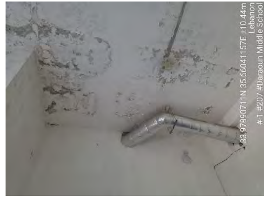
Figure 14- Water leakage
