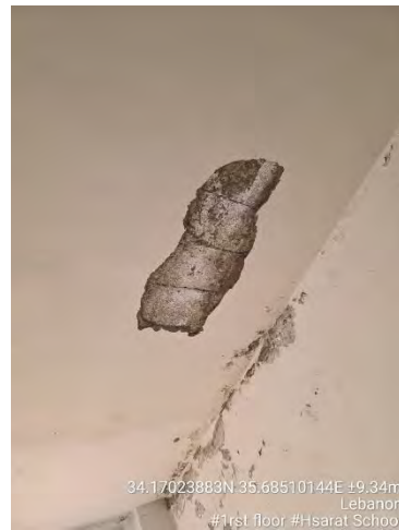
Figure 12- Damaged Plaster
