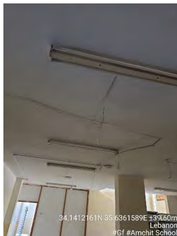
Figure 7- Damaged Lighting Fixtures
