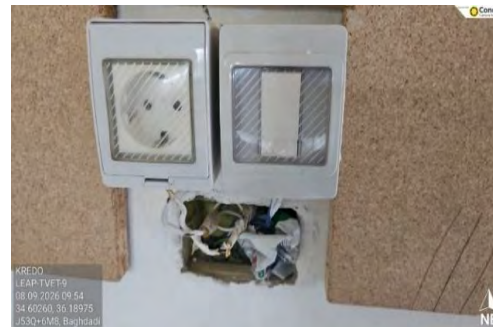
Figure 12- Damaged Socket
