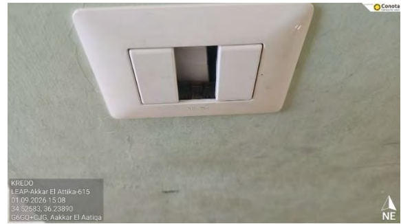
Figure 9 – Damaged Socket
