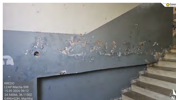
Figure 10 - Water leakage
