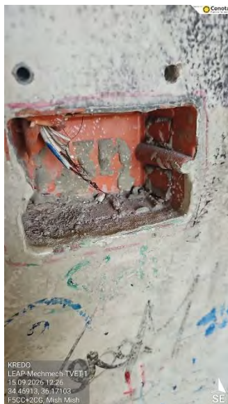
Figure 15 - Damaged sockets
