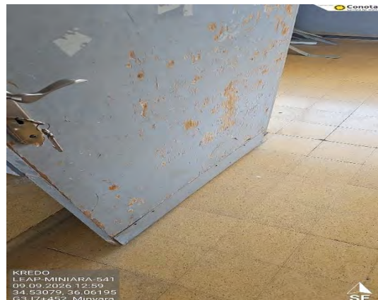
Figure 5 - Damaged door
