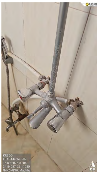
Figure 11 - Damaged mixers
