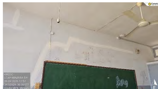
Figure 7 - Damaged paint
