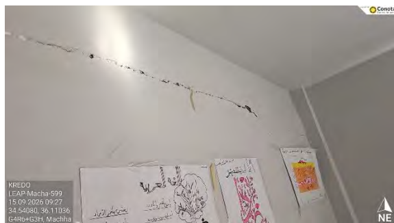
Figure 9 - Wall cracks
