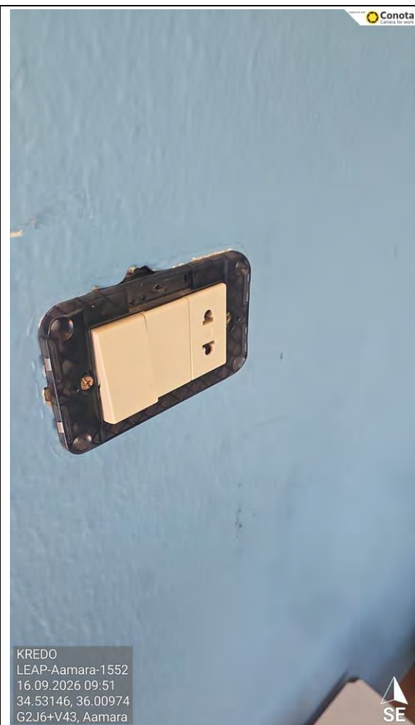
Figure 8 - Missing Socket Cover
