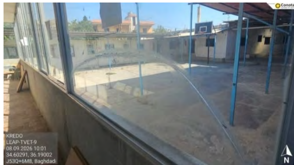
Figure 13- Cracked Glazing
