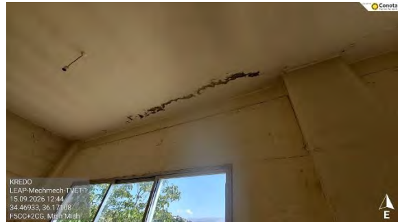
Figure 14 - Water Leakage
