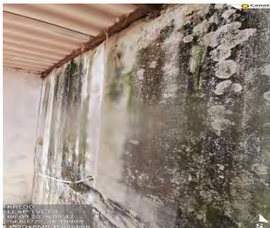
Figure 11- Water Leakage
