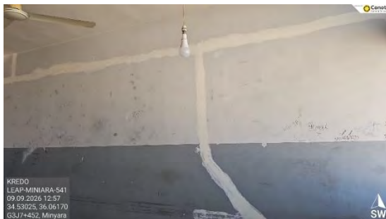
Figure 6 – Wall cracks
