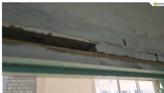
Figure 17 - Damaged plaster
