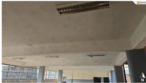
Figure 8 – Damaged Paint
