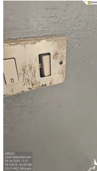
Figure 11 - Damaged switches
