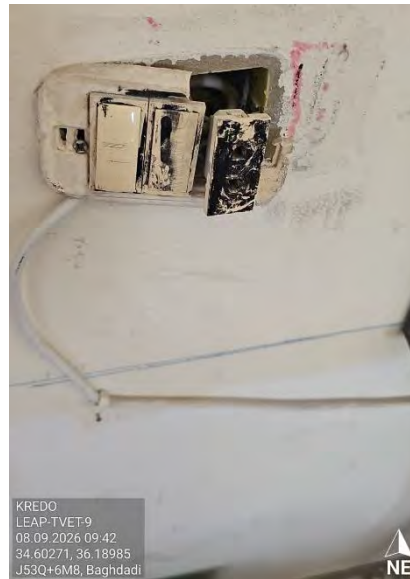
Figure 14- Damaged Switches
