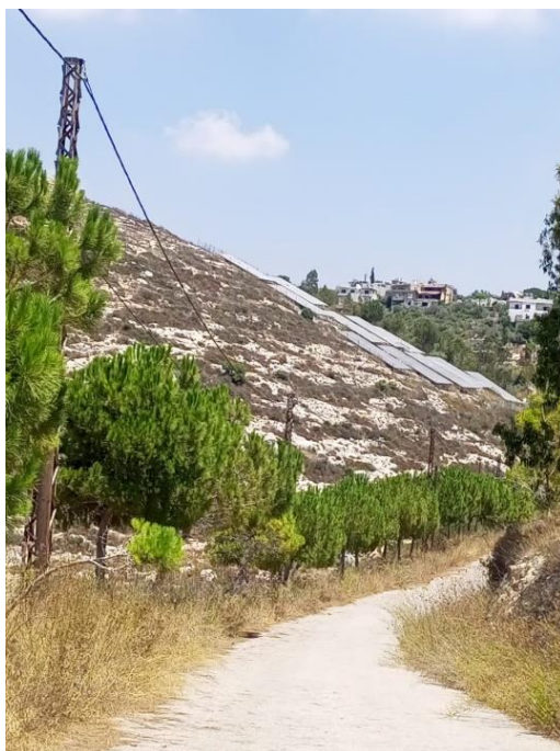
S2-5 — solar PV panels damaged near the pumping station
