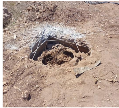
S2-1 / S2-4 — destroyed well head and network from well head to station/reservoir
