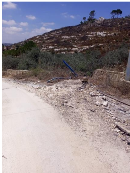
S2-1 / S2-4 — destroyed well head and network from well head to station/reservoir
