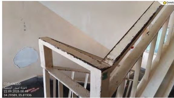
Figure 17 - Rusted Handrail
