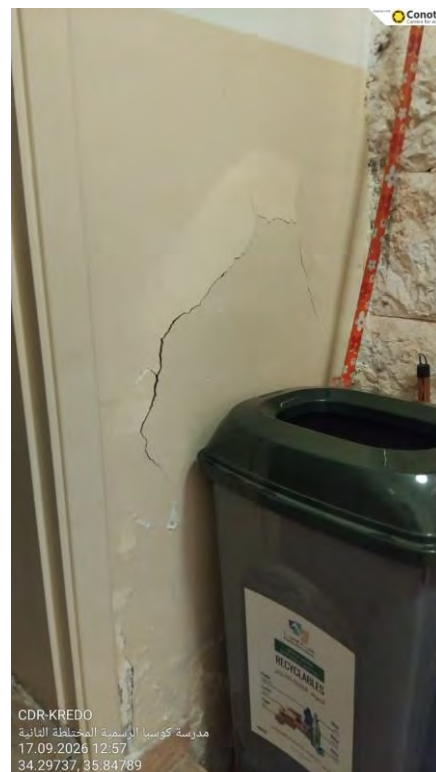
Figure 13 - Damaged Plaster
