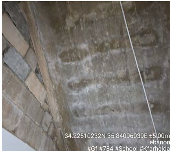
Figure 5- False ceiling collapse due to using the toilets for shower
