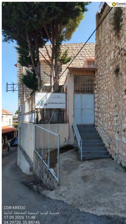
Figure 8 - Door to Playground
