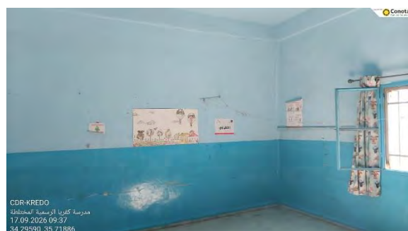
Figure 9- Walls to paint
