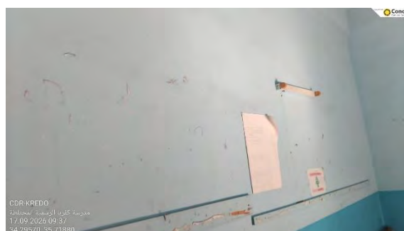
Figure 8- Walls to paint
