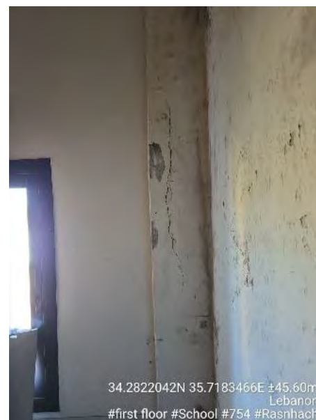
Figure 8- Column crack
