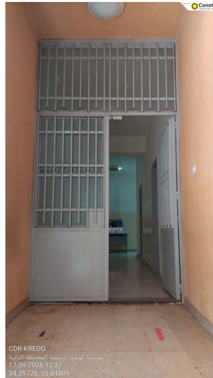
Figure 11 - First Floor Gate
