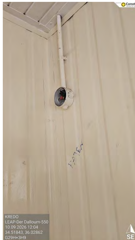
Figure 5 - Damaged socket
