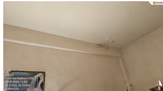
Figure 9 – Water leakage
