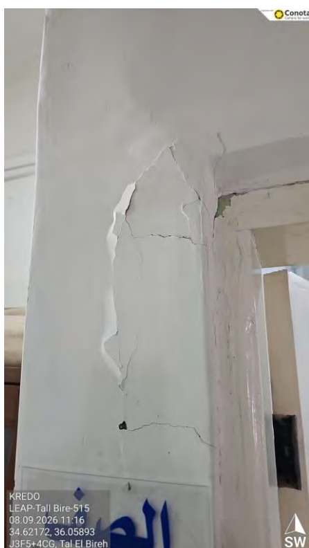
Figure 6 - Wall cracks
