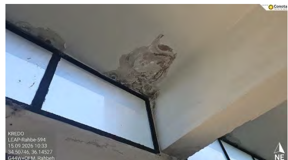
Figure 10 - Water leakage
