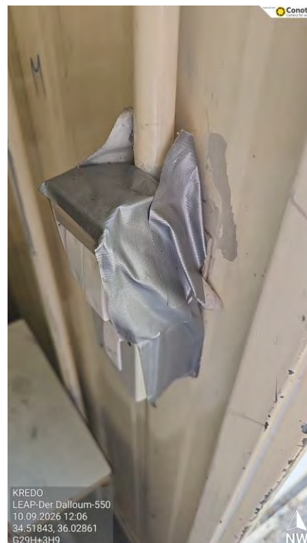
Figure 13 – Damaged switches
