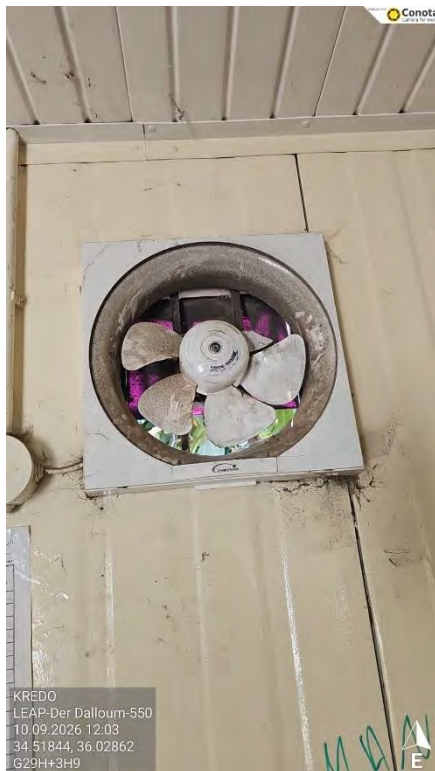
Figure 4 – Damaged fan
