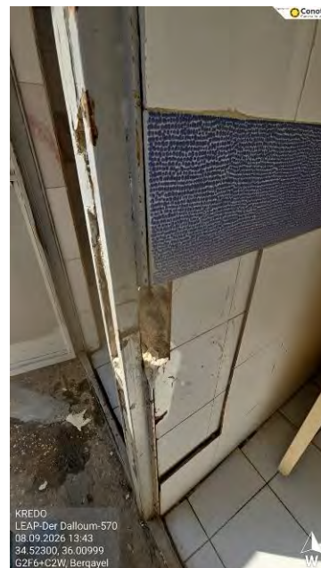
Figure 11 - Damaged Tiles
