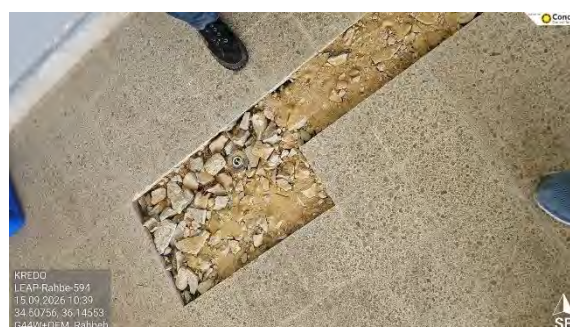
Figure 16 - Damaged tiles
