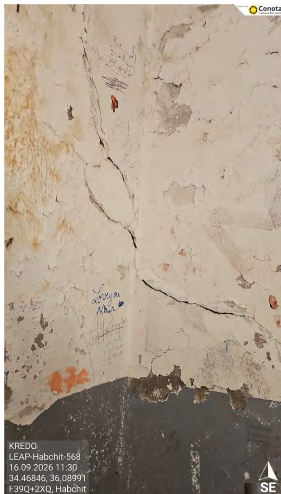
Figure 11 - Wall Cracks (1)
