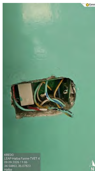
Figure 12 – Damaged Socket
