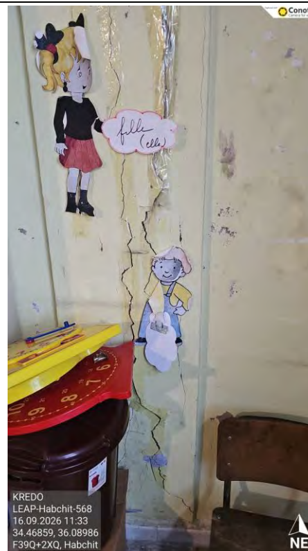
Figure 8- Column Cracks (2)
