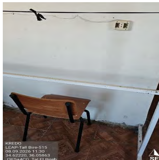
Figure 9 - Damaged socket
