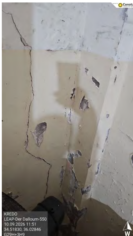
Figure 6 – Wall cracks
