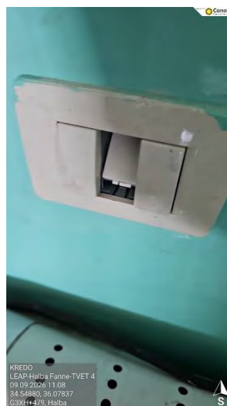
Figure 14 – Damaged Switches
