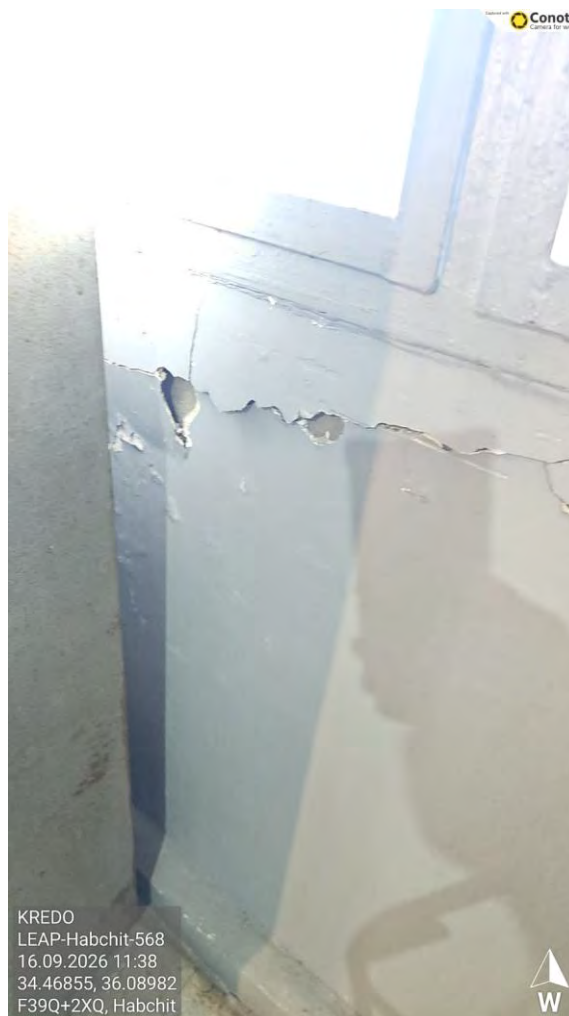
Figure 12 - Wall Cracks (2)
