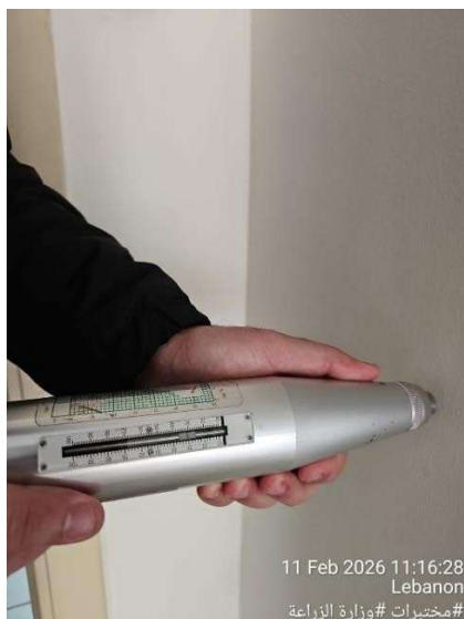
Schmidt hammer test on RC Columns
