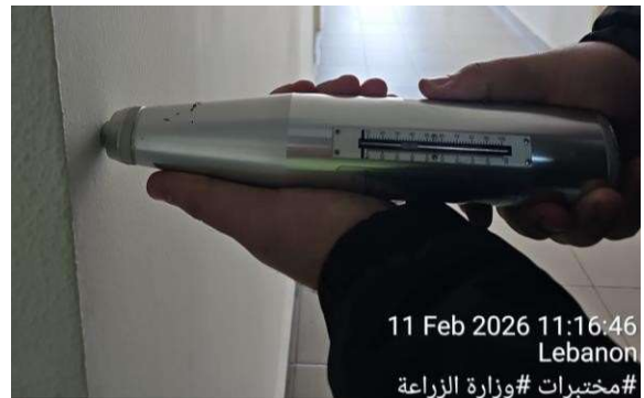
Schmidt hammer test on RC Columns
