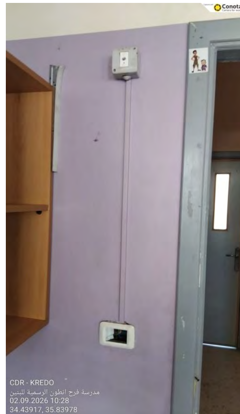
Figure 7 – Damaged Switches
