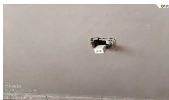
Figure 13 – Damaged Socket
