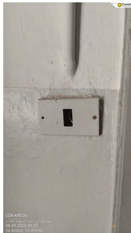
Figure 11 – Damaged Switch
