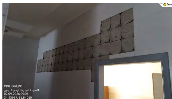
Figure 13 – Missing Tiles
