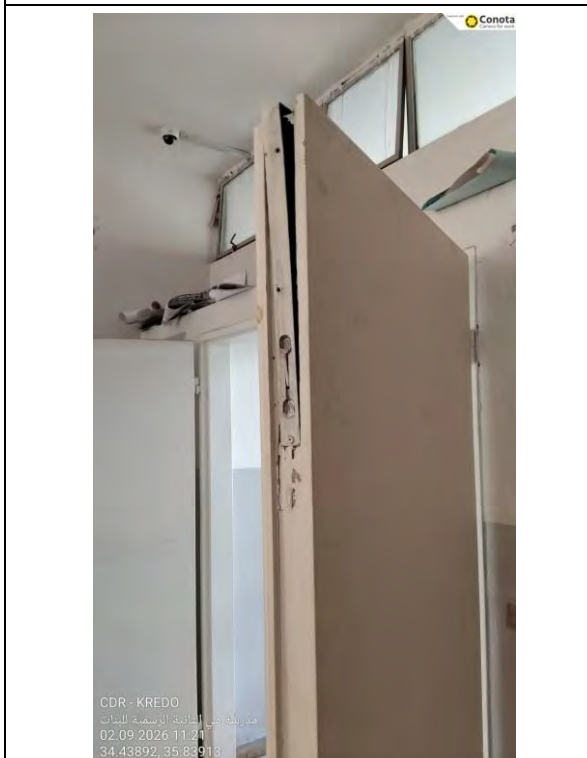
Figure 8 – Damaged Door
