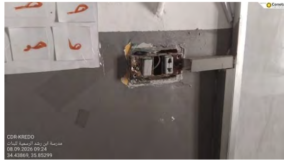
Figure 12 – Damaged Switch
