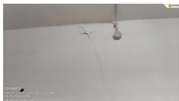
Figure 10 – Plaster Defects
