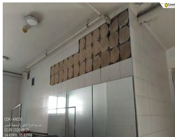
Figure 19 - Missing Tiles
