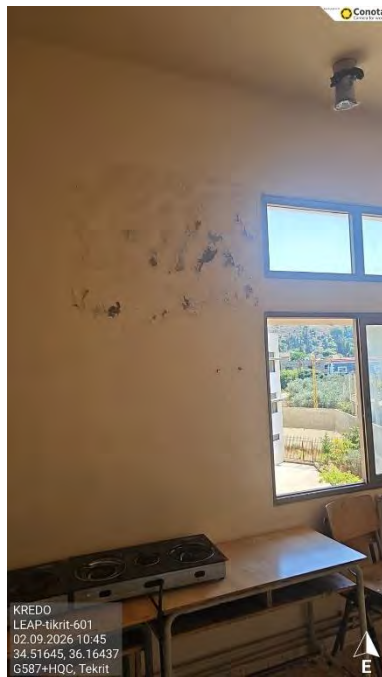
Figure 4 – Water Leakage
