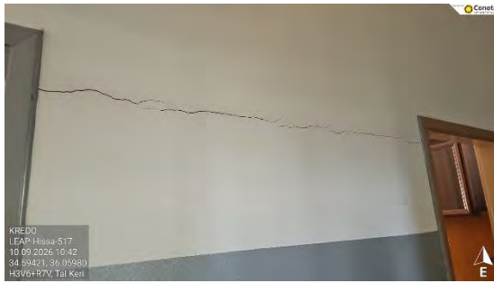
Figure 4 – Wall Cracks
