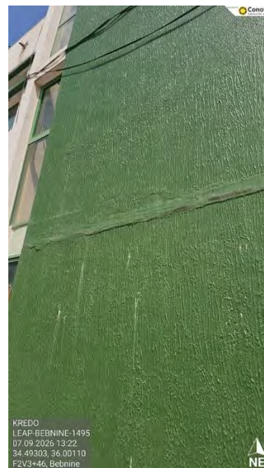
Figure 7 – Facade cracks
