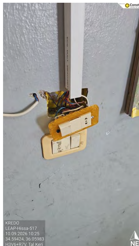
Figure 9 – Broken Socket
