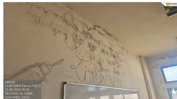
Figure 14 - Water Leakage
