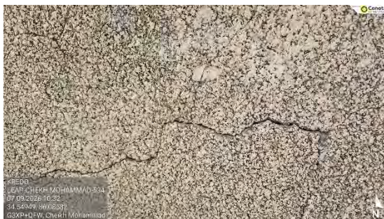
Figure 6 - Façade Cracks
