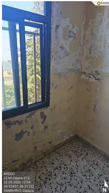
Figure 4 – Water Leakage
