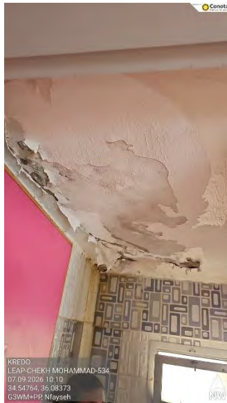
Figure 4 - Water Leakage
