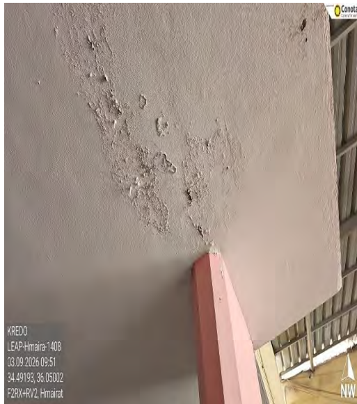
Figure 4 – Water leakage
