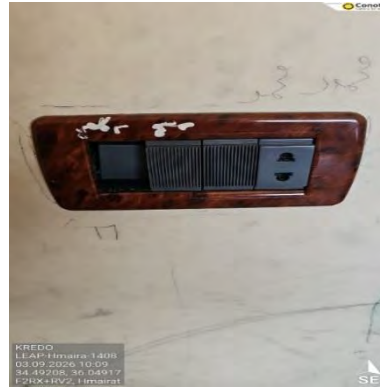
Figure 9 – Damaged socket
