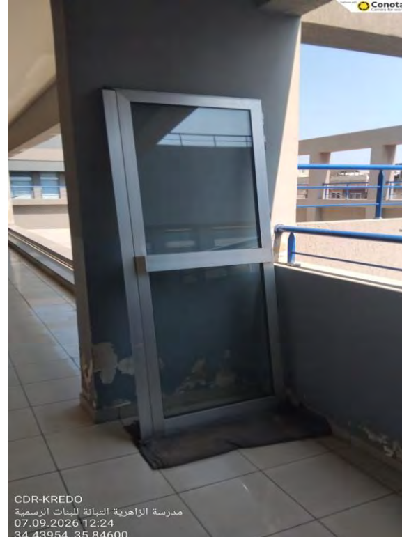
Figure 10 – Aluminum Door to be Installed
