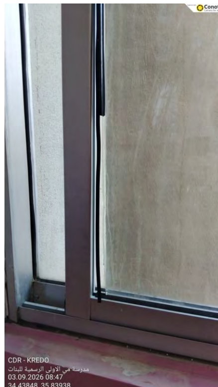
Figure 9 – Broken Glazing
