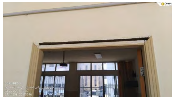
Figure 13 – Missing Architrave
