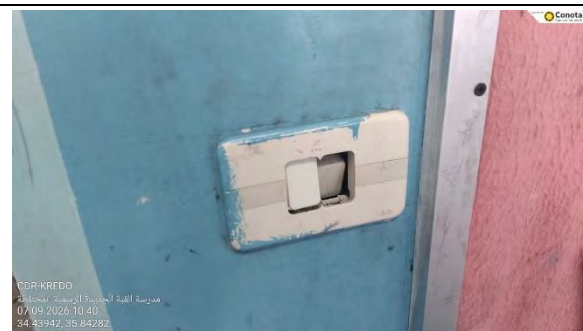
Figure 8 – Damaged Switch
