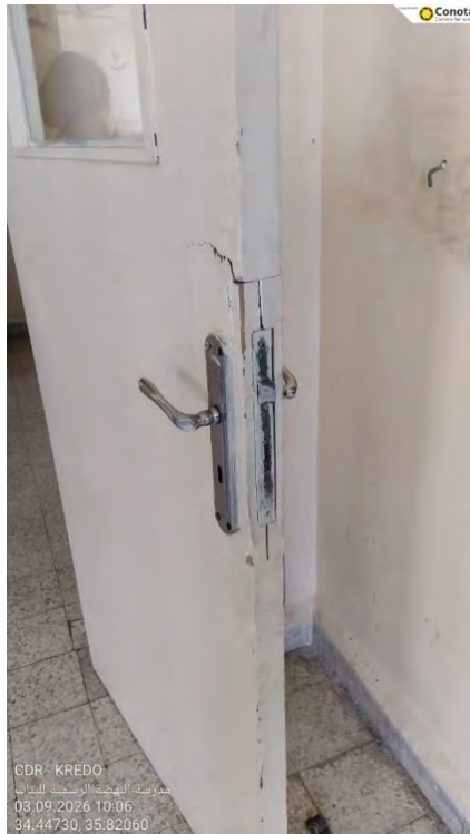
Figure 12 - Broken Door
