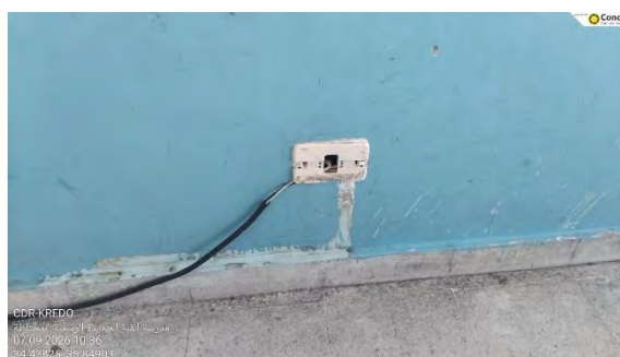
Figure 19 - Damaged Socket
