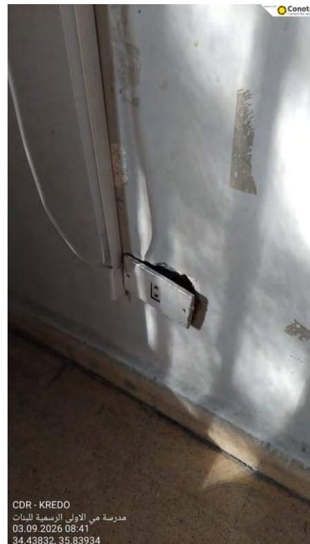
Figure 7 – Damaged Socket
