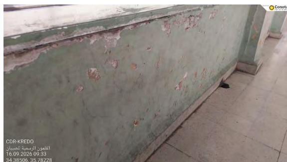
Figure 13 – Damaged Wall
