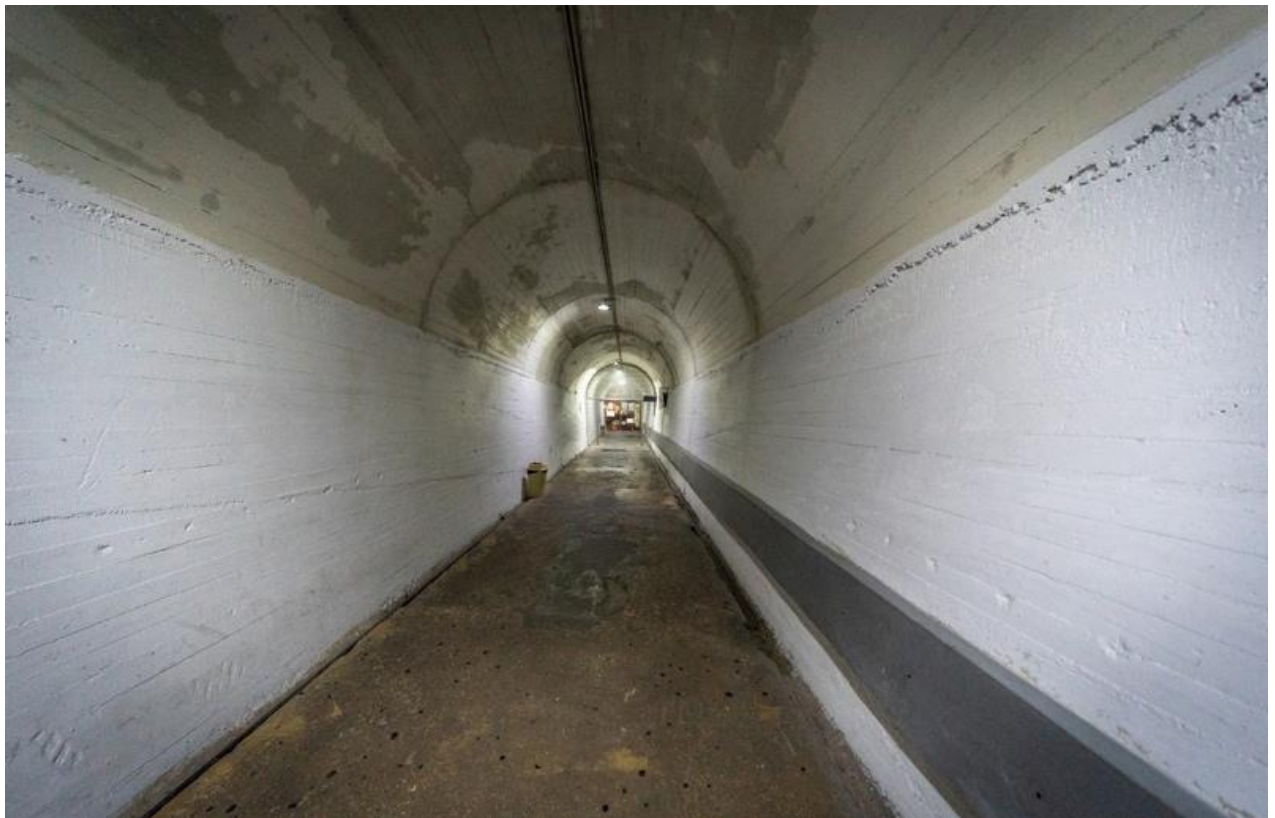
Figure 4 - 117 m Concrete Tunnel Entrance to the Upper Grotto
