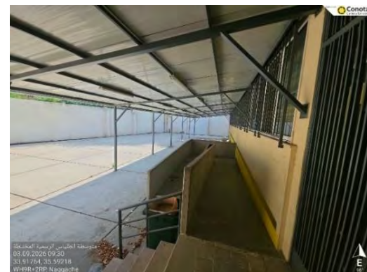
Figure 7- Accessible ramp in good condition
