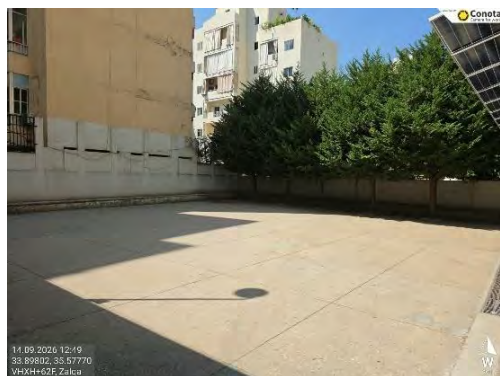
Figure 8- Damaged paint facade
